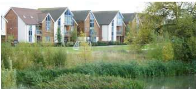
Subtle variation of dwelling typologies and materials overlooking attenuation basin. Limited use of materials palette to emphasise development character.
