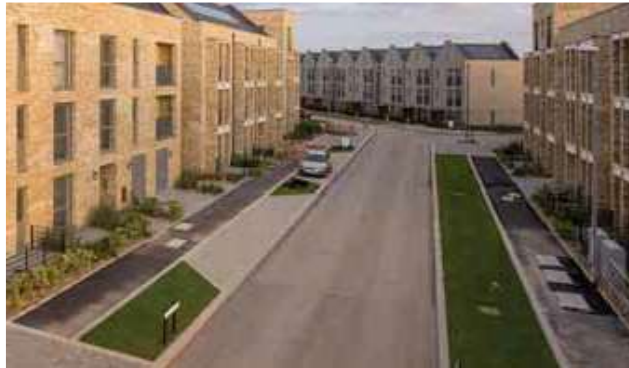
Figure 38 Consistent building line
