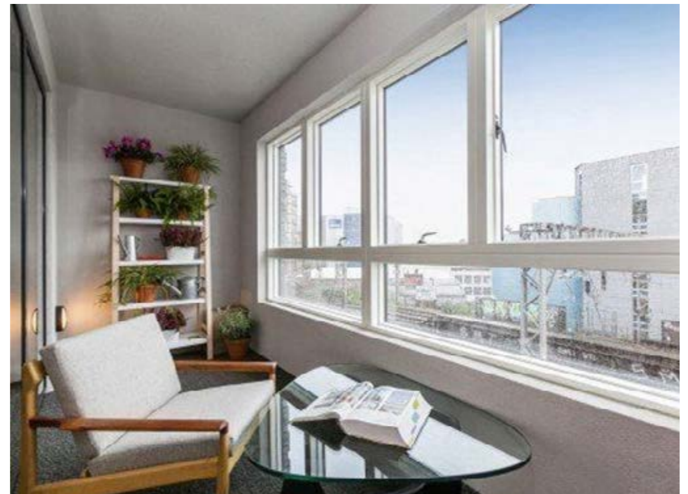
Mint Street, Bethnal Green by Pitman Tozer Architects Wintergardens provide a habitable buffer from an adjacent trainline.
