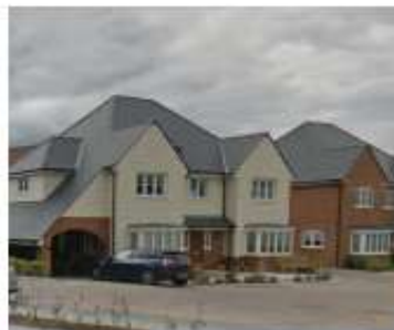
Variation in roof scape and building materials within same street scene
