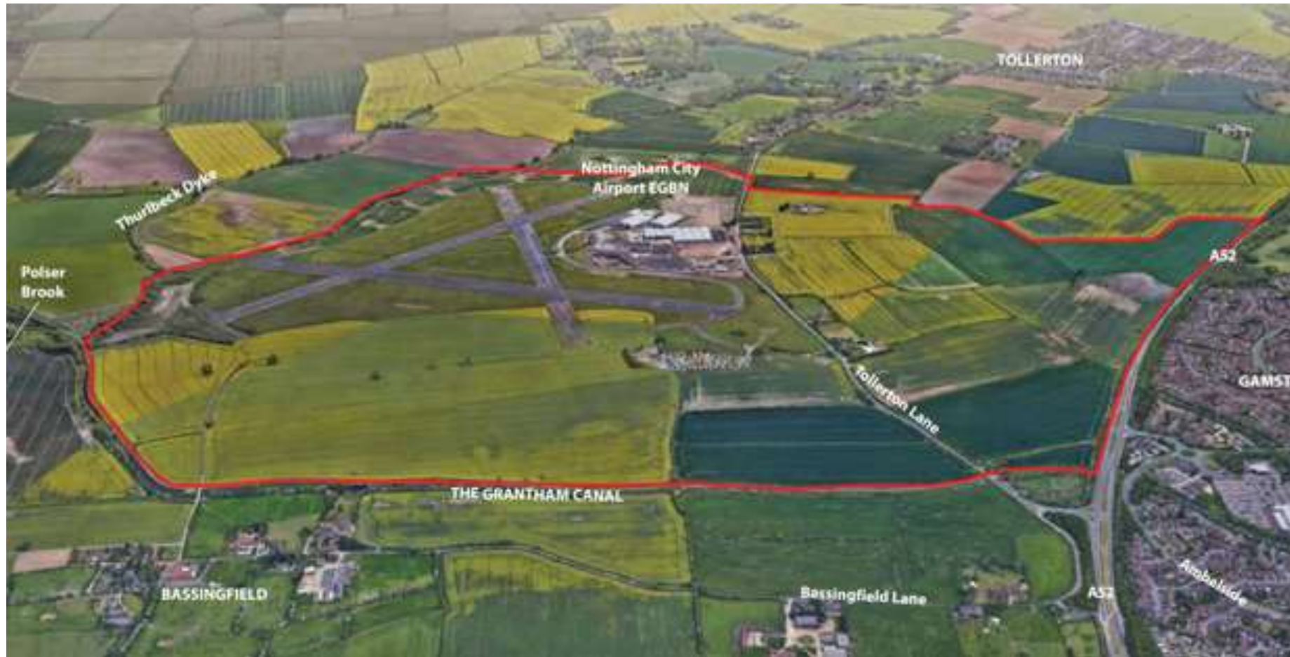
Figure 3. Aerial view looking south over of Strategic Allocation Site
