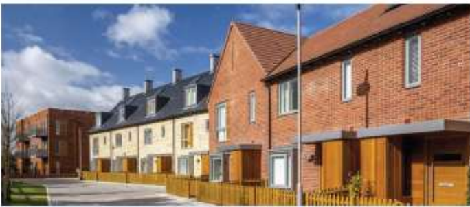
Occasional change of roof profile and materials. Common elevation features repeated throughout same street scene.
