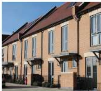
Building form and massing with symmetrical rhythm to create a formal and urban character.
