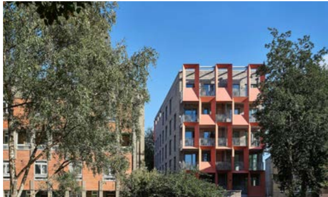
Orwell House, Tower Hamlets, London by Bell Philips uses an ornamental frame/shade articulate the mid-rise of the apartments.
