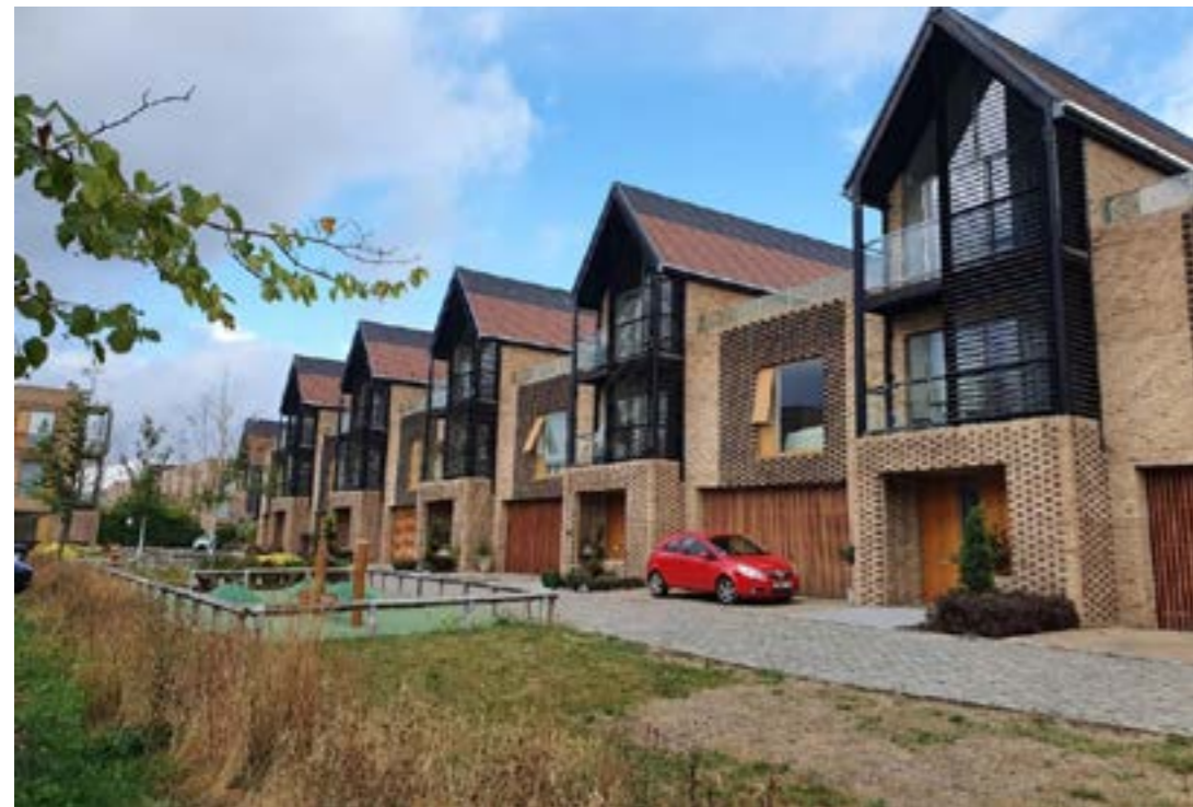
Ninewells, Cambridgeshire, Tertiary street with doorstep play and linear park (Photograph by Rebecca Clark)
