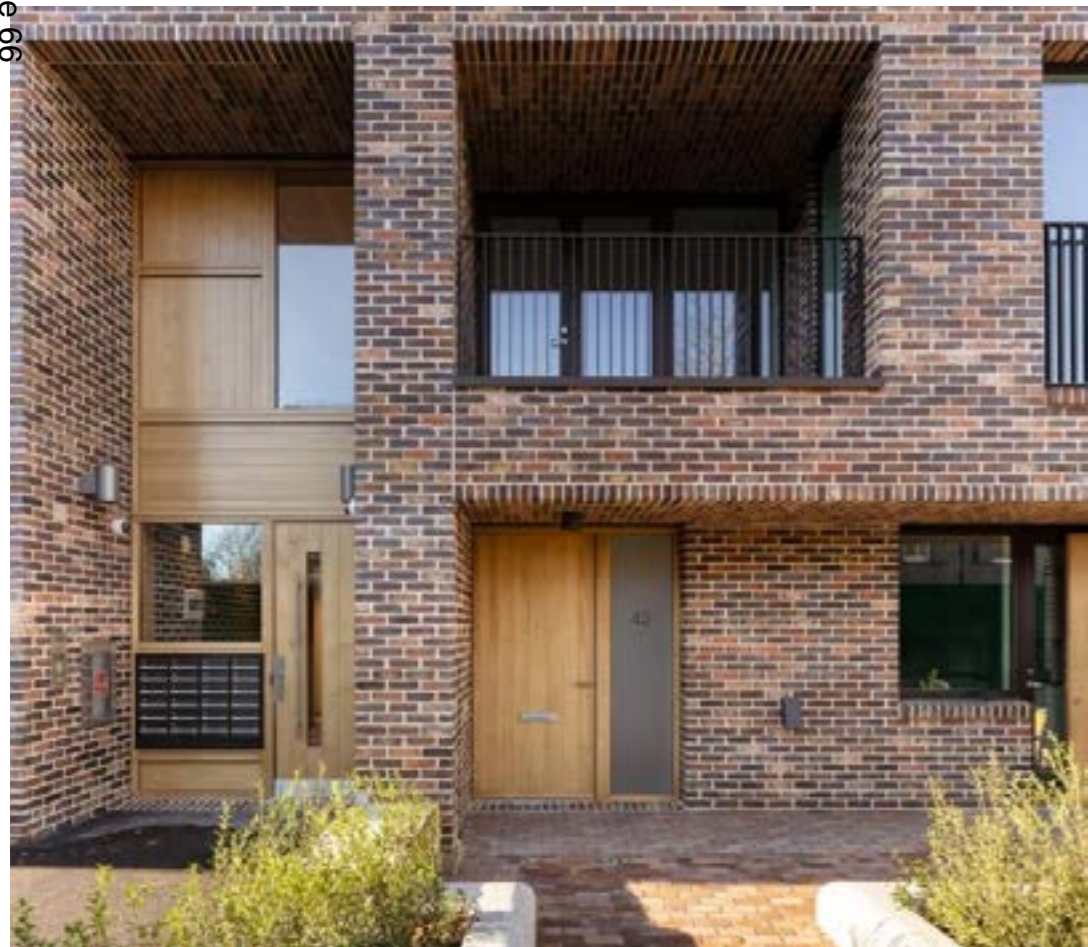
Branch Place, Colville Estate by Karakusevic Carson Architects. Communal entrance is generous and clear (left of image). Private residential doors provide further ground floor activity (right of image)
