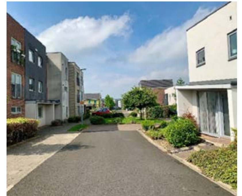
Staithe housing, Gateshead. Street designed for walking speeds. Varied planting creates a buffer between houses and street, whilst clear visibility of entrances and front windows help animate the street. (Photographs by Rob Beardsworth)
